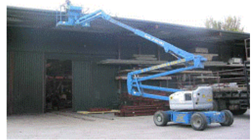
Using a MEWP to clean a gutter
