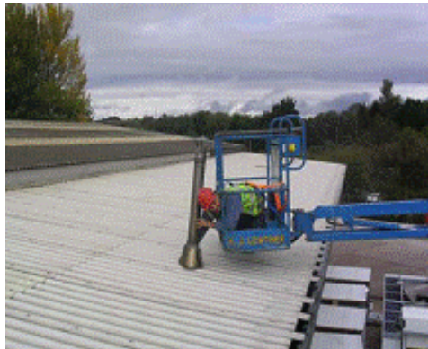
Using a MEWP to inspect a vent
