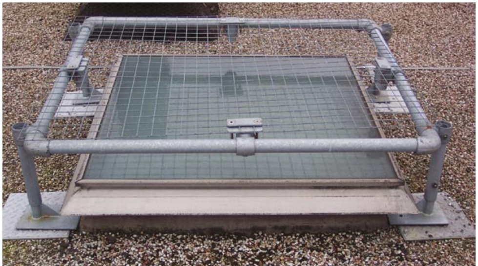
Covers can be fitted to existing roofs or included as part of the design (Image courtesy of Safesite)
